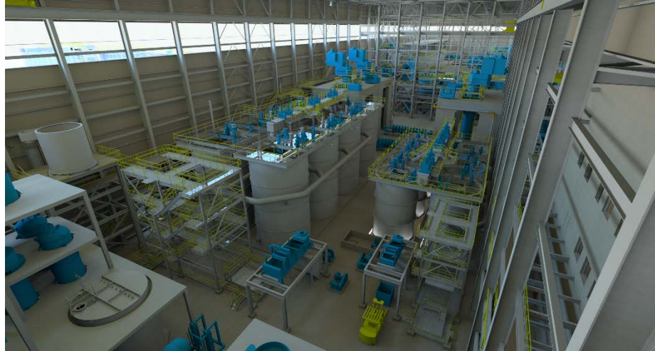
Figure 17-12: Configuration of the CIP and gold recovery circuits
