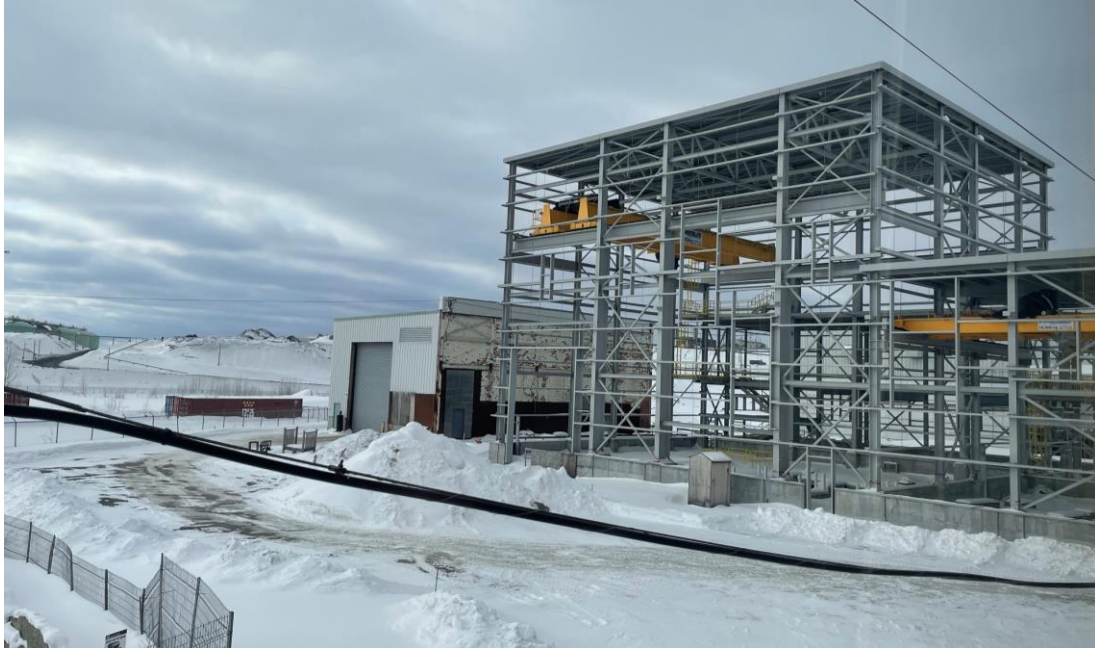
Figure 12-1: Unfinished hoistroom at the Quemont site (February 2021)
