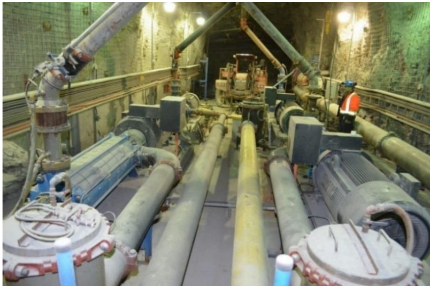
Figure 16-26: Typical underground multistage pump dewatering station
