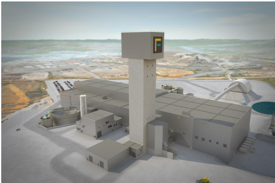
Figure 18-6: Headframe and hoist room buildings
