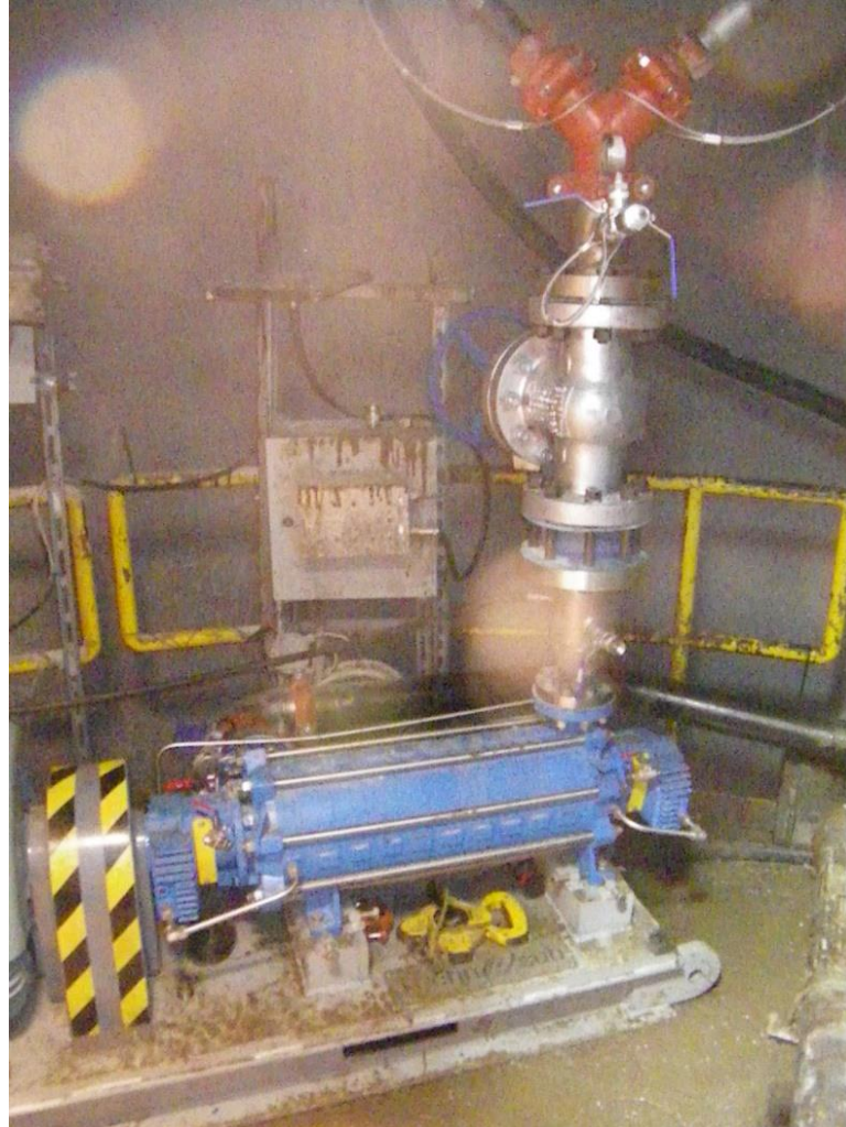
Figure 16-13: Typical booster pump installed on a Galloway
